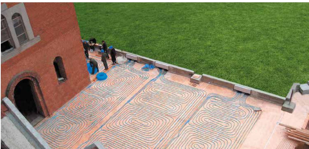
Att. 5. Heating installation of outdoor patio employing KAN-therm system bluePERT pipes.
